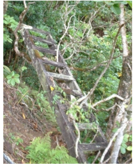
Remnant of wooden ladder. Photo by John M. Flanigan
