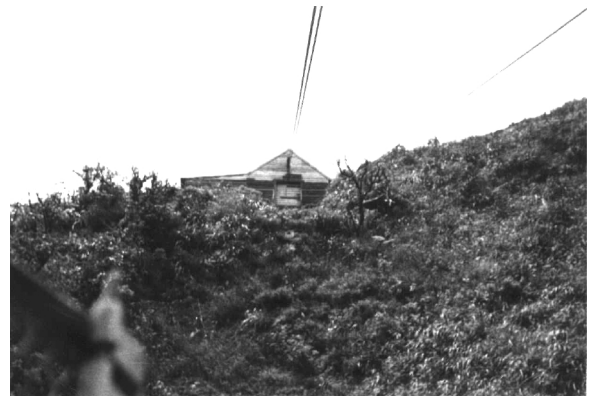
The tramway cage docked at the upper hoist house as seen from the stairway. Photo by David W. Jessup, 1946
