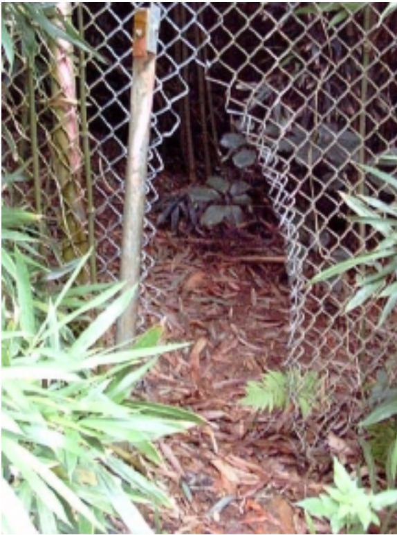
Vandalism of perimeter fence provides illegal access. Photo by John M. Flanigan
