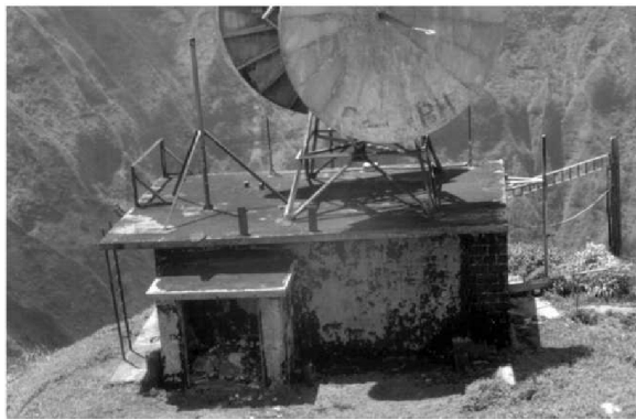
Helicopter view of the Communication Control Link building, c. 1960. From the collection of the Ha‘ikū Omega station.
